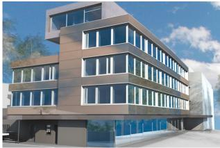
The addition of a storey to the existing office building at Lessingstrasse 3 in Zurich proved to be a challenge, but Timbatec solved it in a well thought-out manner. Today, the building presents itself with two additional floors in timber construction. Here 5 new apartments were created.
