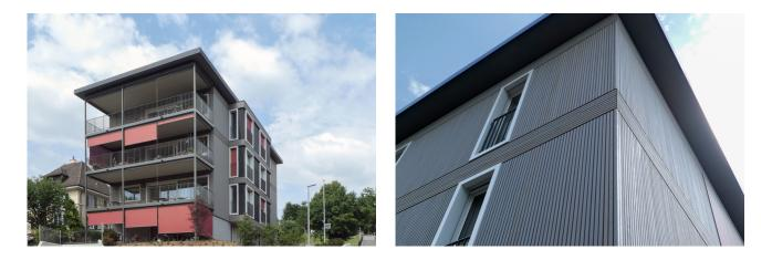
In the case of the apartment building on Zürichstrasse in Küsnacht, practically everything that protrudes from the ground is made of wood. The building, which is located in the middle of the Zurich suburb, comprises four apartments with a view of Lake Zurich.
