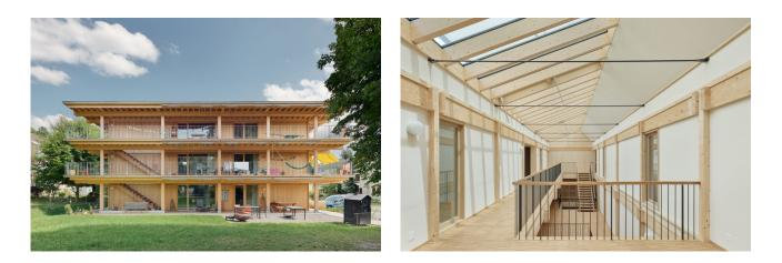
In the Generationenhaus Mooseggstrasse, a lot of beetle wood and almost no glued cross-sections are used. The skeleton construction is part of the architectural expression.
