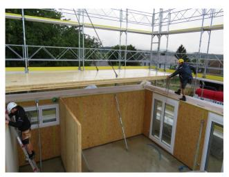
Assembly of CLT panels on the construction site
