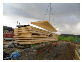
Delivery of CLT panels to the construction site
