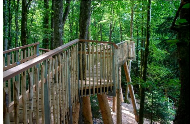
The 25-meter-long treetop walkway adds another attraction to the forest playground in Ballenberg. The platform stands up to 9 meters high on round logs. Timbatec prepared the structural analysis for this project.
