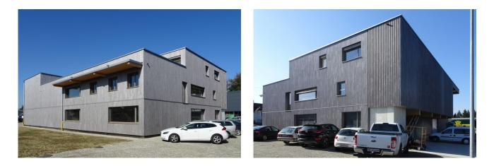
In Aefligen, between Bern and Solothurn, a commercial building with various ancillary rooms was built. The building with a volume of over 6,000 cubic meters convinces with its load-bearing structure and the facade made of wood.
