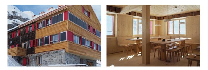
The Lämmerenhütte of the SAC was extended by five meters. The building material was flown to the hut by helicopter.
