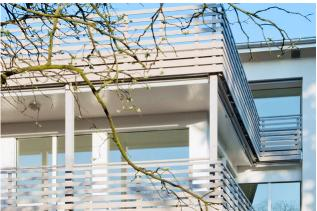
The existing apartment building on Salvatorstrasse underwent a total renovation to create more space, comfort and aesthetics. The living room extension consists of hollow box elements, which rests on a post and beam construction at the front and is clad with a glass front.
