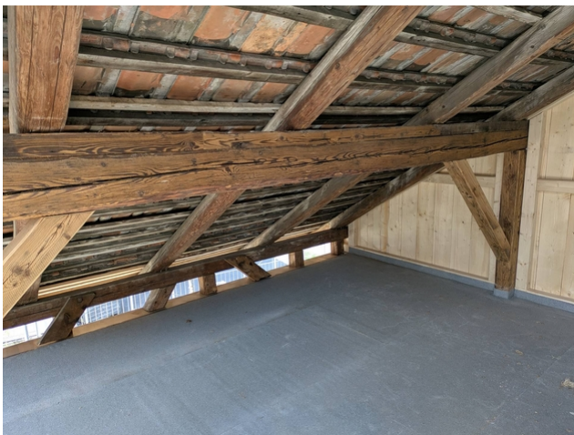
Reinforcement of the existing roof structure with reclaimed wood.
