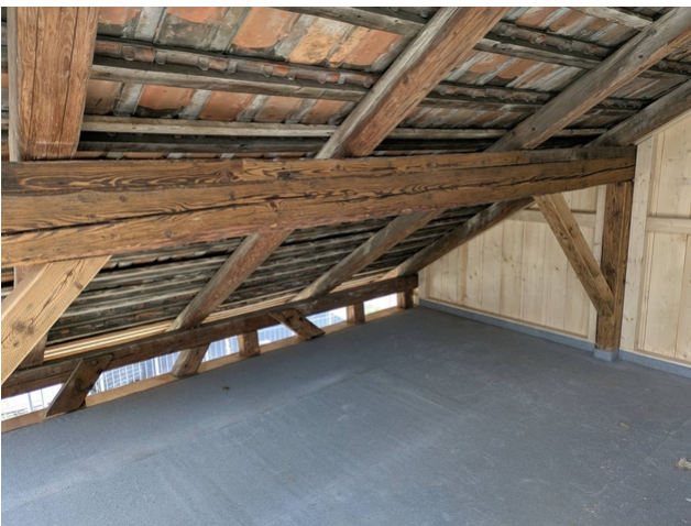
Reinforcement of the existing roof structure with reclaimed wood.
