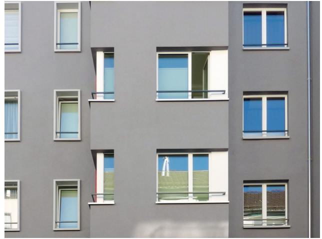
Bay window finished
