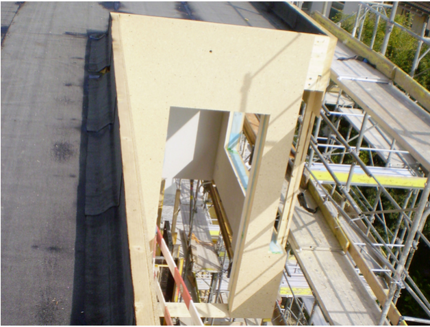
Addition of storey carcass
