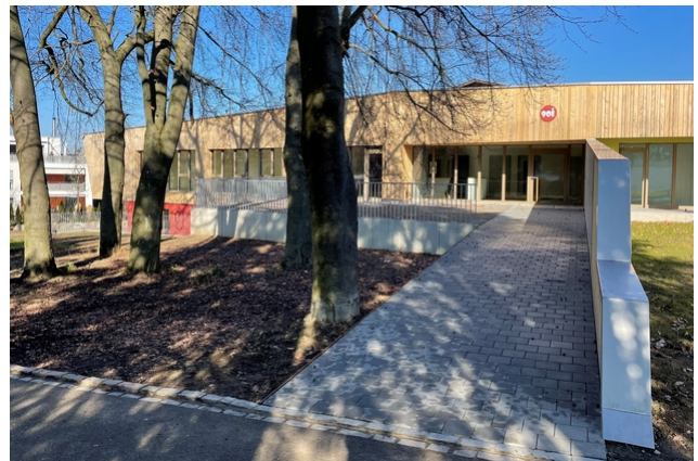
Construction and facade are made of wood
