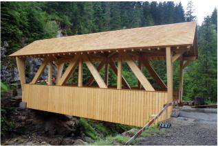
The bridge connects the districts of Sense and Gruyères and received a certificate for the use of Swiss wood. The new truss structure with shingle roof replaces the old Höllbach bridge, which was destroyed by arson in 2013.
