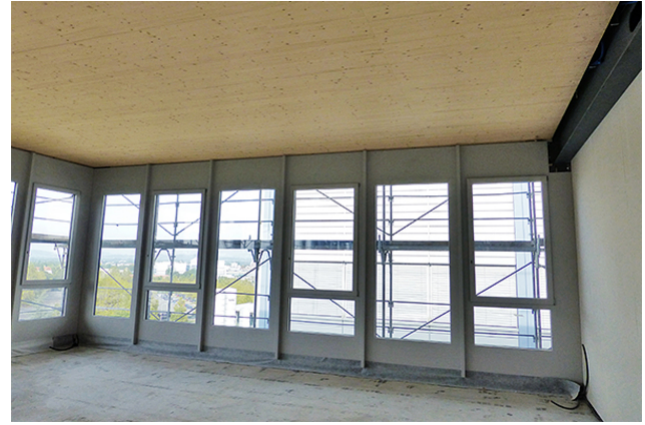
Wooden ceiling with 9m span
