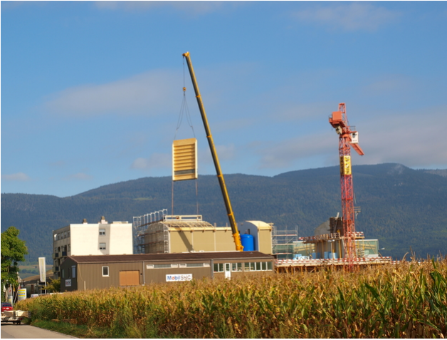
Assembly exterior walls
