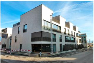
The four-story wooden building stands on the eastern outskirts of Bern. Thanks to recesses and inwardly offset balconies, small areas are created that make the object with dimensions of  $37 \times 16 \times 12$  m appear smaller and break up the silhouette.
