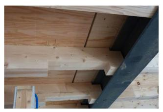
Cutouts for building services installations in the rib elements of the floor slabs
