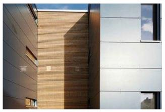
In a picturesque, elevated location on the south-western slope of Wohlen, this 6-family mini-house was realized in timber construction. The apartments are arranged as two-flats on both sides of the staircase and built in pure timber construction.
