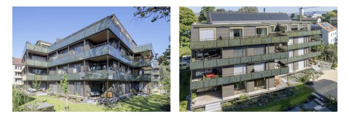
The new replacement buildings in Zurich Altstetten are among the first projects that can do without concrete in the stairwell as well. This has been possible since the revision of the fire protection guidelines in 2015.
