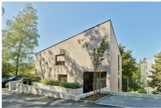
The apartment building in Kilchberg is completely built in wood, including staircase. The special feature: The wooden outer wall of the first floor is half buried in the ground.
