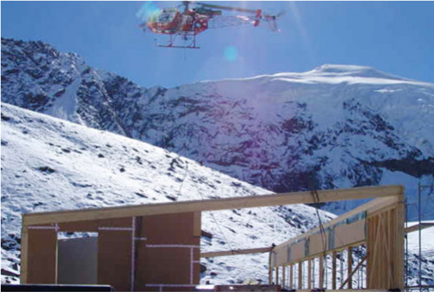
Erection with helicopter
