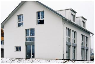
The client planned to build a spacious housing estate in Ottenbach in wood. The aim was to create a reference for modern buildings in optiholz board stack construction.
