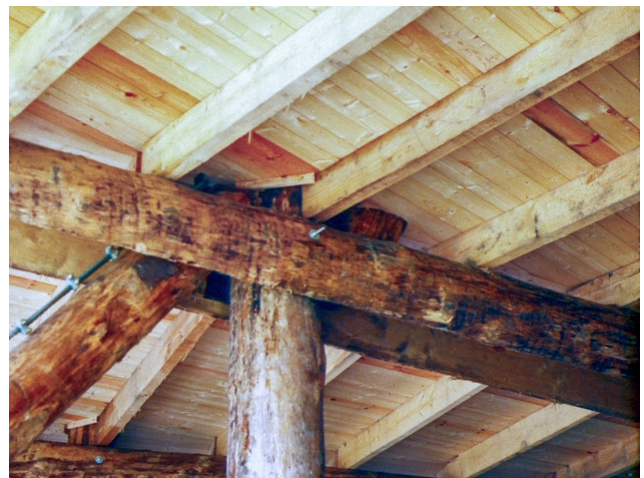
... and the application on the construction
