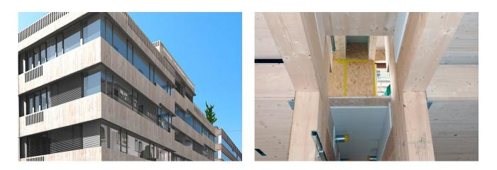
An exciting new building project on Habsburgstrasse in Zurich. A 5-storey MFH as a pure timber construction. Solid construction despite difficult fire protection conditions. The central staircase core and the fire wall to the neighboring building brace the column-slab construction.
