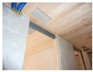
Wall coating as a heat accumulator
