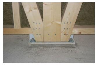
Anchoring earthquake bracing
