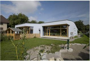
The new double kindergarten in Uttigen was planned and executed as a pure timber construction. The building should have a simple and inexpensive construction. The use should also remain variable - school meetings should also be able to take place there.
