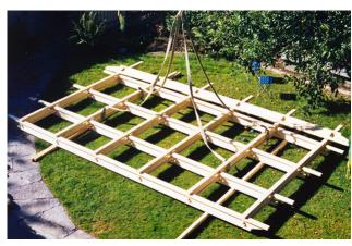
Fold out girder grid on flat surface and install edge and reinforcement girders
