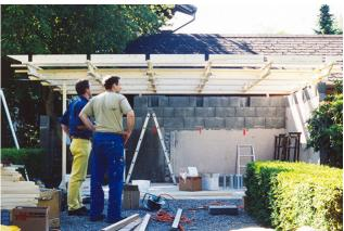
The client was looking for a solution for the roofing of their seating area. They wanted a more unusual solution than purlins and rafters. The situation allowed 2 line supports on 2 masonry walls at right angles to each other and a point support on a pendulum support.
