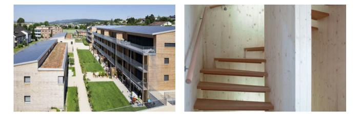
The development in the Minergie-P Eco standard is designed as a zero-energy housing estate and consists of 2 multi-family houses and 7 terraced single-family houses. The entire settlement is built from the first floor in timber construction.
