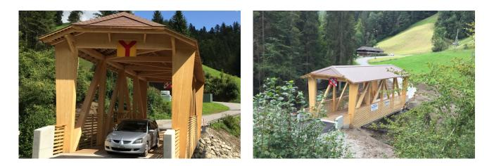
The new wooden bridge connects the two Bernese villages of Horrenbach-Buchen and Teuffenthal near Thun and replaces an old concrete bridge. The new crossing is capable of carrying loads of up to 32 tons.
