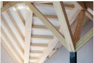
In the most beautiful location directly on the Wohlensee, a sophisticated single-family house was built in Hinterkappelen. On the massive basement, a building with three floors was erected in timber construction. The wall elements were realized in timber frame construction. A board stack construction was chosen for the floor slabs. Generous galleries, high rooms and a lot of window area characterize the modern building.
