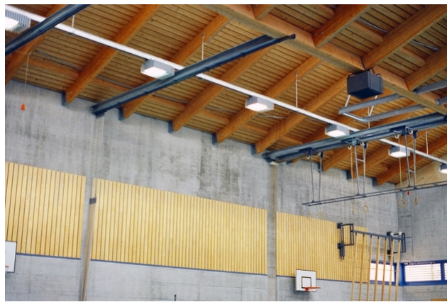
View of exposed rafter position
