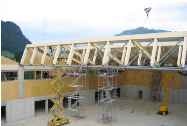
Assembly of lattice girders
