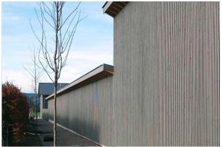
The Polo Park Zurich has relied entirely on wood as a building material for its new center. Both the operations building and the various stable buildings with the horse stalls have been realized as timber frame buildings.
