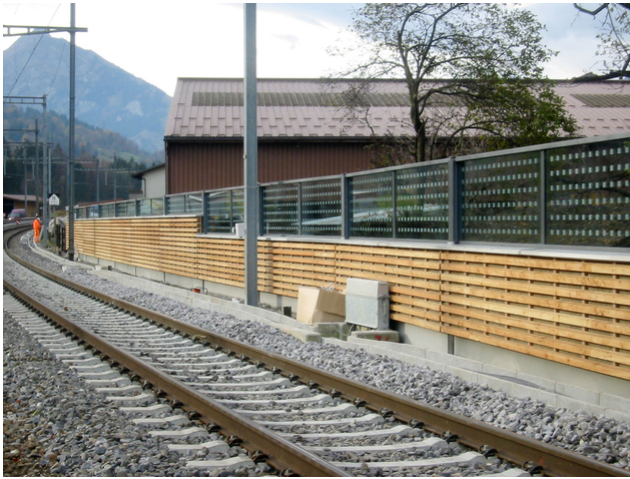
View from the track side
