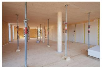
During the curing of the casting resin, the floor slabs must be additionally supported
