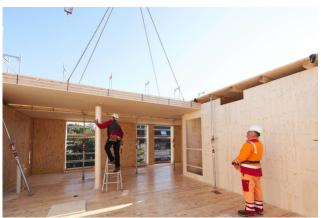
In Frenkendorf, the first four-story column-and-slab structure made of wood was built. Thanks to TS3, the building once planned in concrete can be built in wood. The planning with the multi-axial load-bearing cross laminated timber panels is similar to reinforced concrete.
