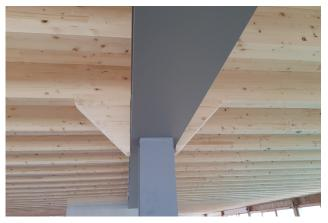
Combination of steel structure and wood construction
