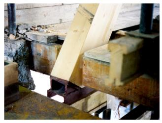
UNP beam, end support truss
