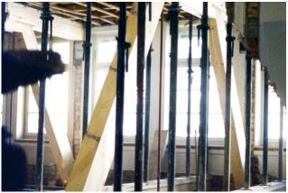
The existing building in the center of Thun was converted into business premises and apartments. On the 1st floor, three high reinforced concrete girders were installed, which protruded from above about 70 cm into the clearance gauge. The planned store was to be column-free with a smooth soffit. The existing beam layers were to remain unchanged.
