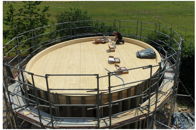
Grouting the TS3 joint
