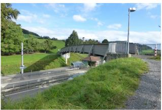
The pedestrian bridge near Vechigen was built in 1999. From the outside it was in relatively good condition, only the upper covers of the main girders seemed weathered and damaged.
