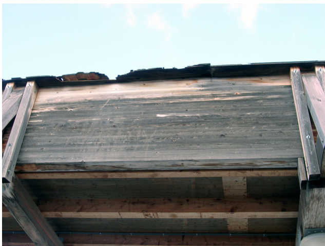
Pedestrian bridge before renovation 2
