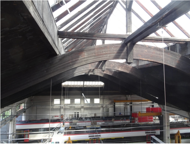
Arch truss with drawstrings
