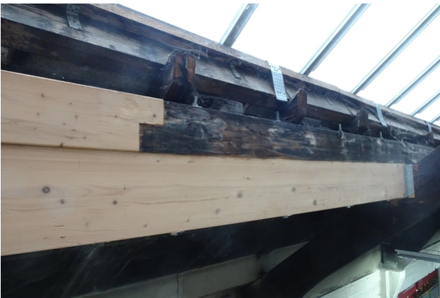
Replacement rafter purlins
