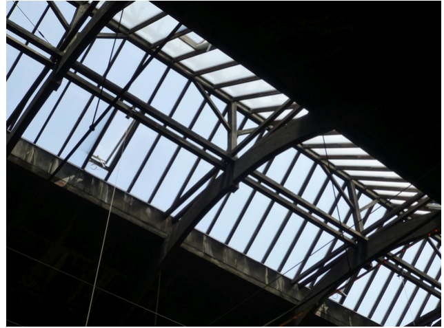
Interior view roof
