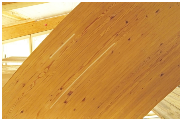
Detailed view of a rehabilitated adhesive joint
