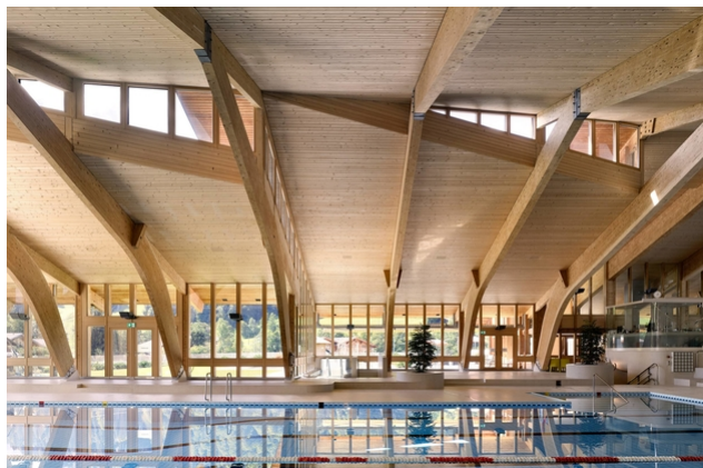
Between the trusses was renewed acoustic paneling
