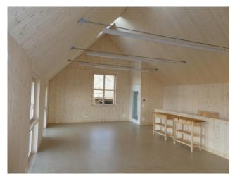
Tie rod for absorbing the static forces
