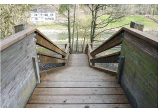
Large parts of the Horgen pedestrian bridge over the Sihltalstrasse had to be replaced. Many central wooden elements of the crossing were in poor condition.
