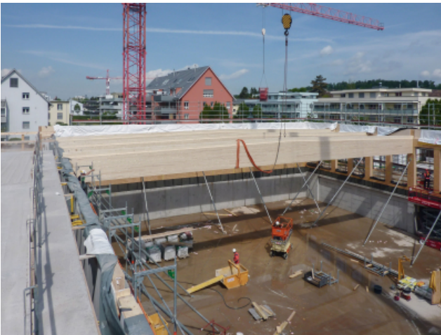
Installation of Roof Racks for the New Gymnasium
