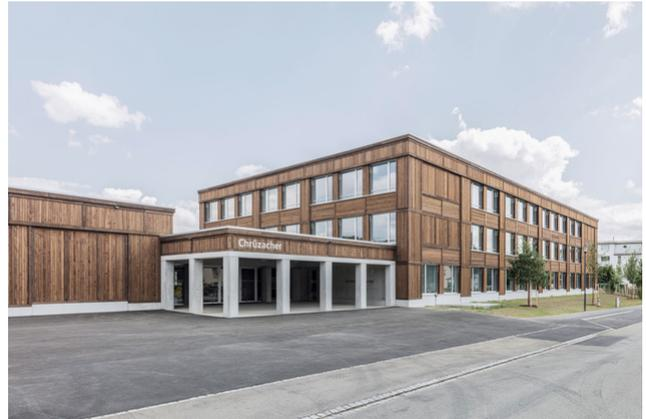
On the initiative of Timbatec, the new school complex in Bassersdorf ended up with even more wood than planned. Originally, only the walls of the gymnasium were to be made of wood, while the roof was to be made of concrete. Timbatec suggested that the roof should also be made of wood in order to save costs.
