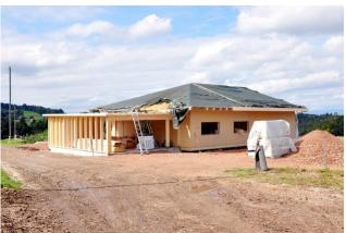
The rurally located single-family house was completely prefabricated and after only 4 months of construction the building was ready for occupancy. The timber construction contains a world novelty - namely the TS 3.0 developed by Timbatec - a ceiling system made of panels, which carry 2-axes analogous to a concrete ceiling.
