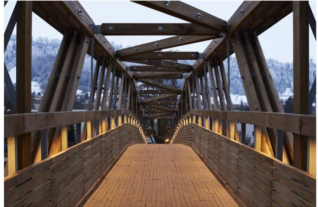
The Tüfisteg pedestrian and bicycle bridge in Adliswil is getting on in years. Analyses showed that replacing the bridge would cost almost as much as renovating it. Today, a new bridge leads over the Sihl - with beech wood from the surrounding forests.
