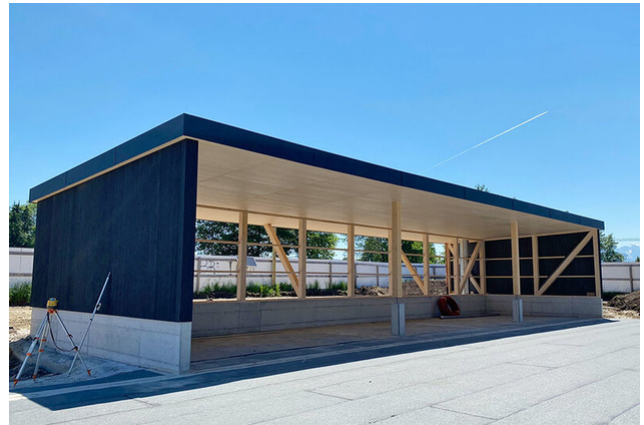
Roofing of the container house
