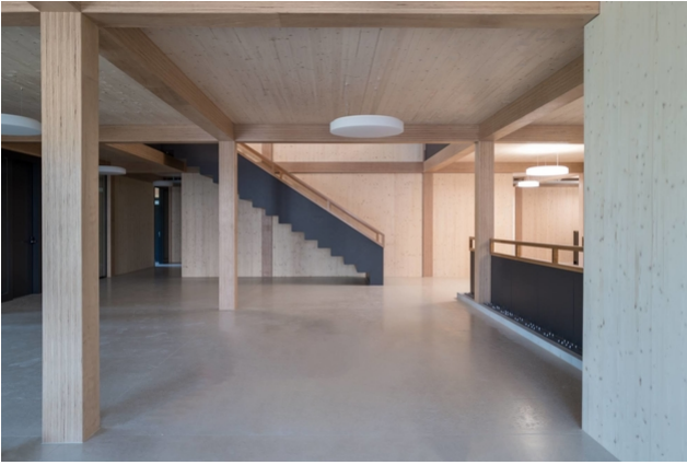
Interior view with beech supports
