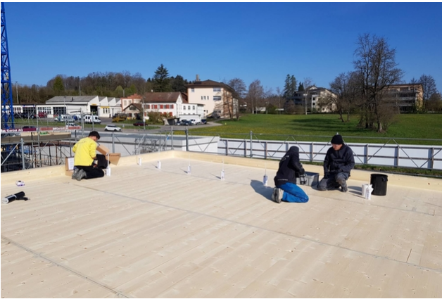
TS3 during TS3 grouting of the canopy
