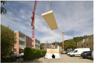
In the middle of the city of Wetzikon in the canton of Zurich, a housing estate was renovated. By adding wooden floors, 36 new residential units were created on top of the prefabricated buildings designed by the architectural icon Ernst Göhner.
