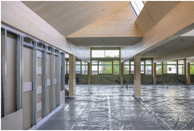
Interior view with wooden construction and acoustically effective Lignotrend ceiling elements
